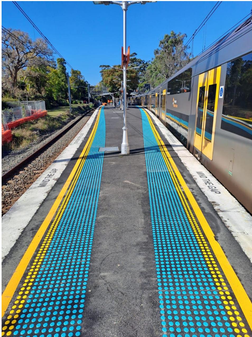
Above: New tactile ground surface indicators on platforms – northern end.
