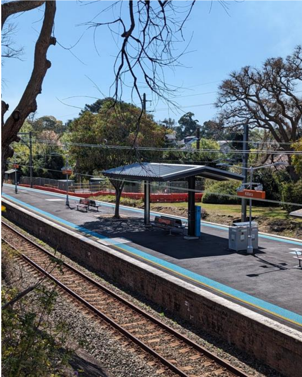
Above: Resurfaced Platform 1 and 2.
