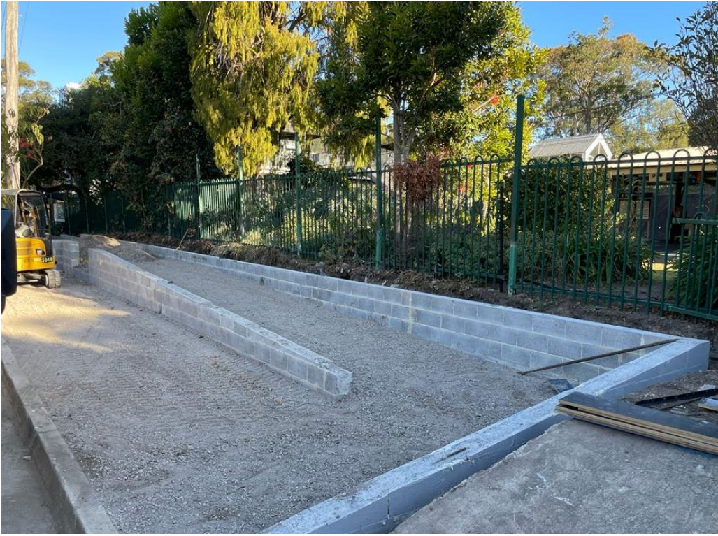
Above: Werona Ave – footpath upgrade
