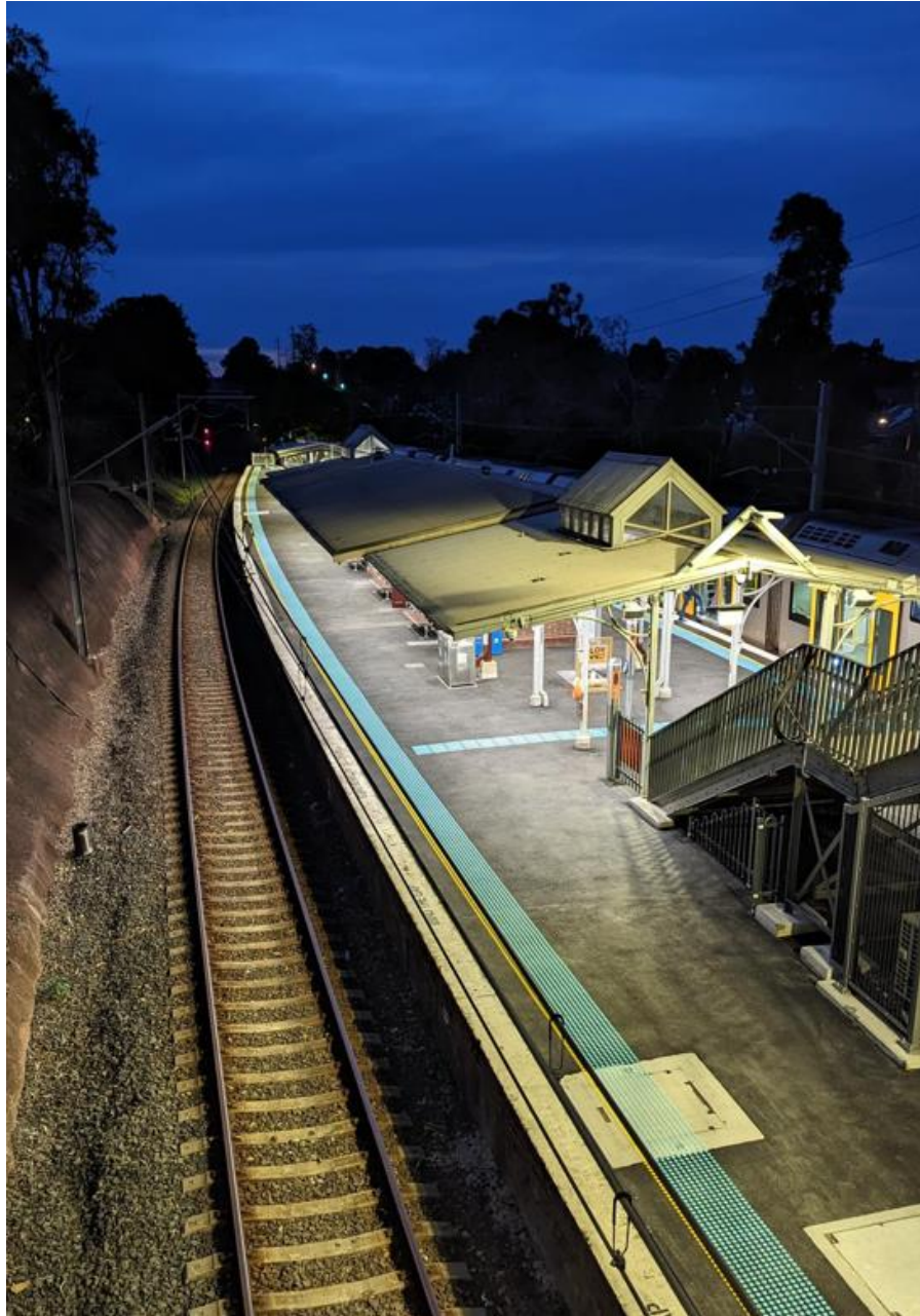
Image: Completed platform resurfacing and installation of tactile ground surface indicators
