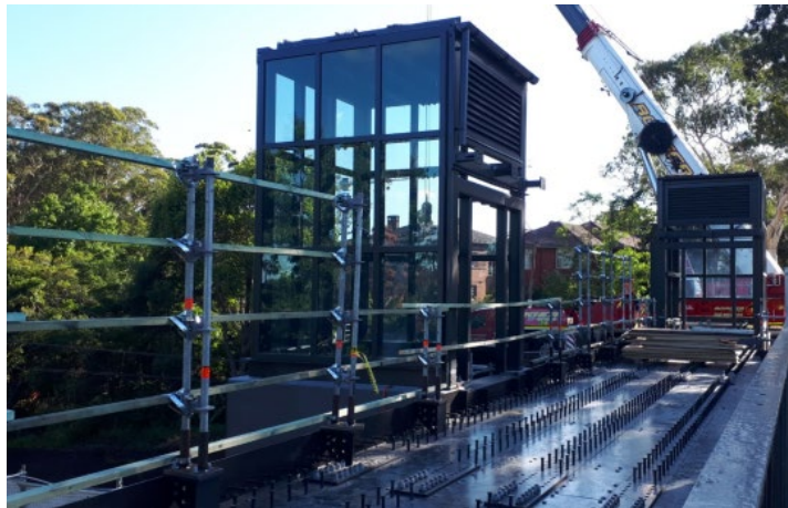
Image showing installation of the structural steel
