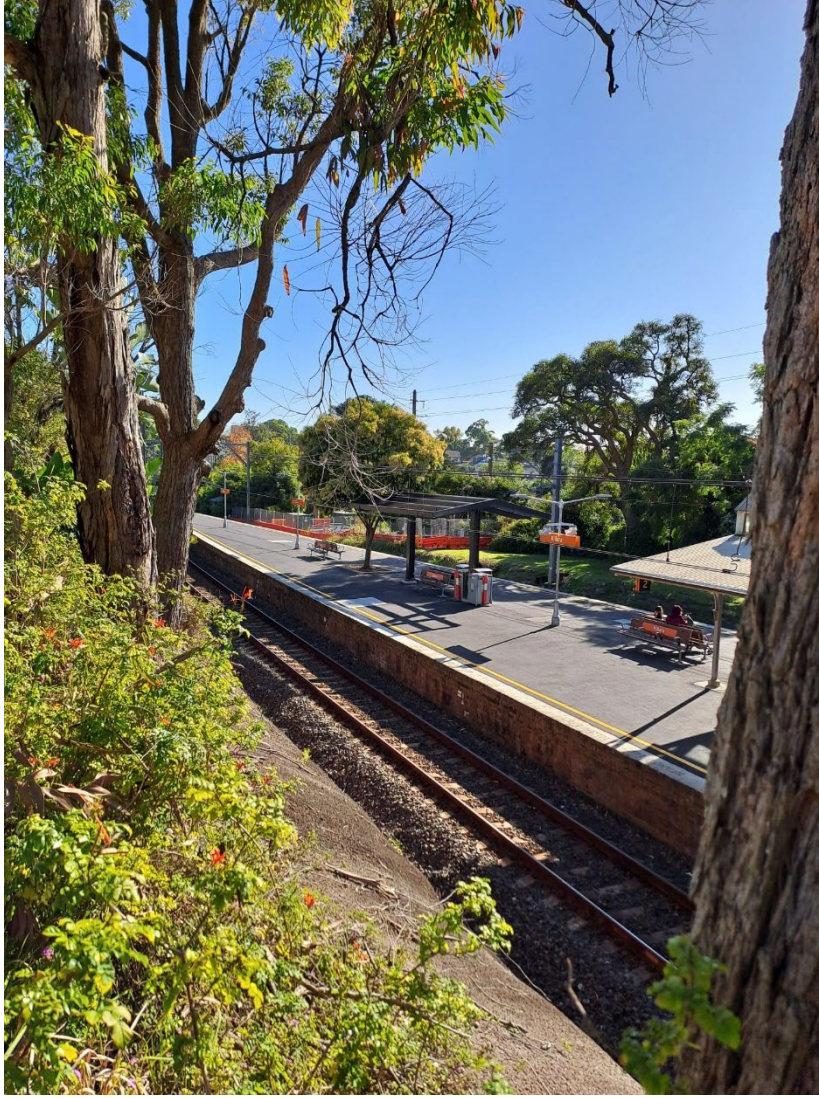
Above: Resurfacing work on the station platform
