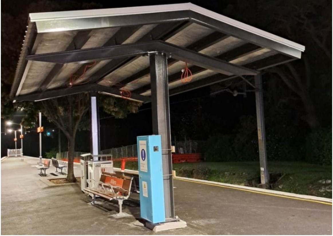
Above: the new canopy for the boarding assistance zone
