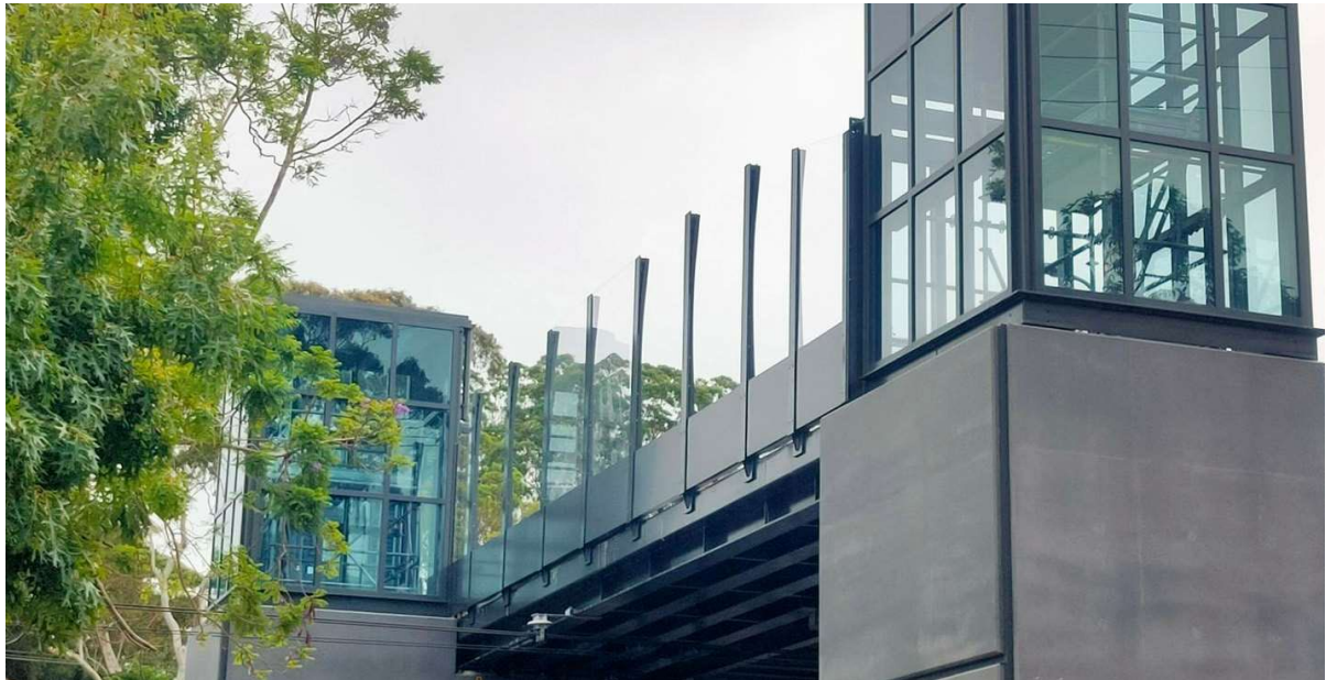
Image above of the bridge screen install at the station
