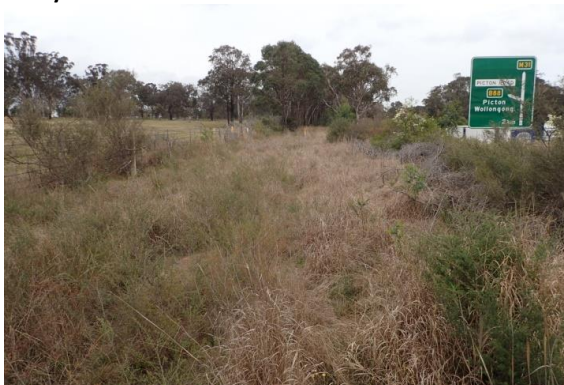
Plate 7. View to south-west. East side of M31, south of Moolgun Creek Bridge. The road reserve included a buried fibre optic cable. Visibility was poor due to grass and shrub cover.
