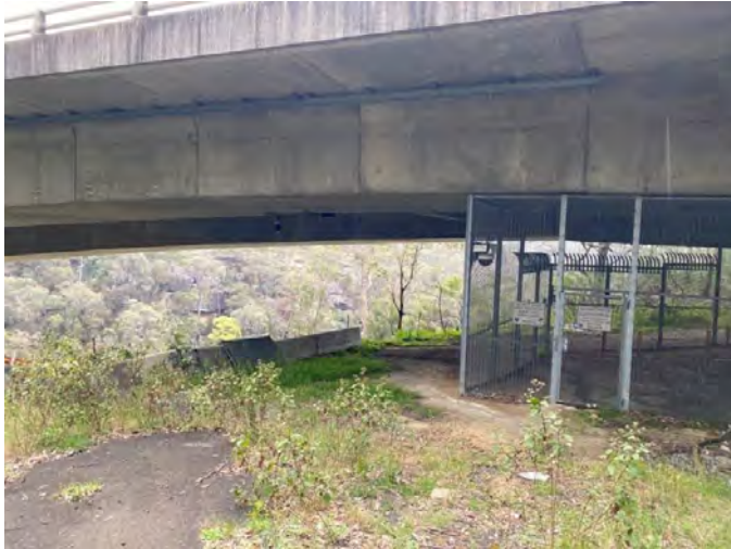
Photo 5-1: Existing crossing under Pheasants Nest Bridge
