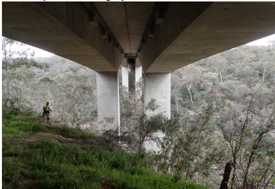
Plate 11. View to south-west at Pheasants Nest Bridge. Under northern abutment.
