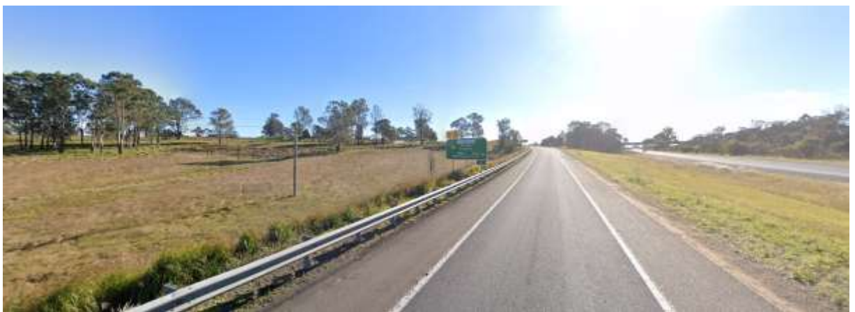
Figure 6-11 Viewpoint 3: Indication of view from nearby residence towards the northbound exit ramp adjacent to Site 3 (Southern Hume) (Image source: Google maps, 2023)
