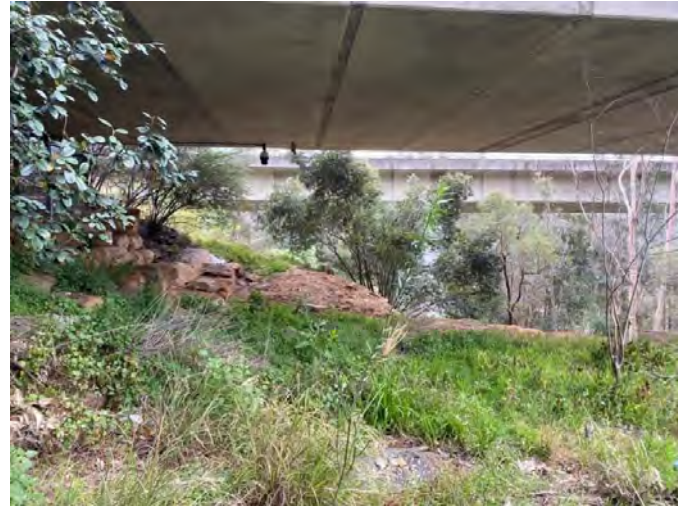
Photo 5-2: Existing crossing under Moolgun Creek Bridge
