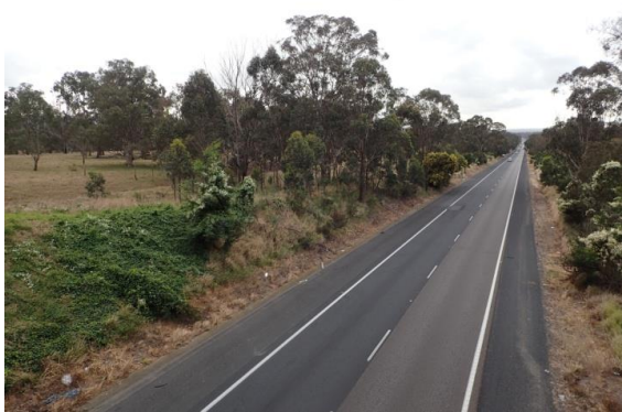
Plate 1. View to north-west. Study area comprised road reserve at left, next to M31 Hume Motorway.
