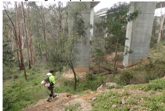
Plate 4. View to north-east. Moolgun Creek Bridge. Western side. Upper valley slopes.
