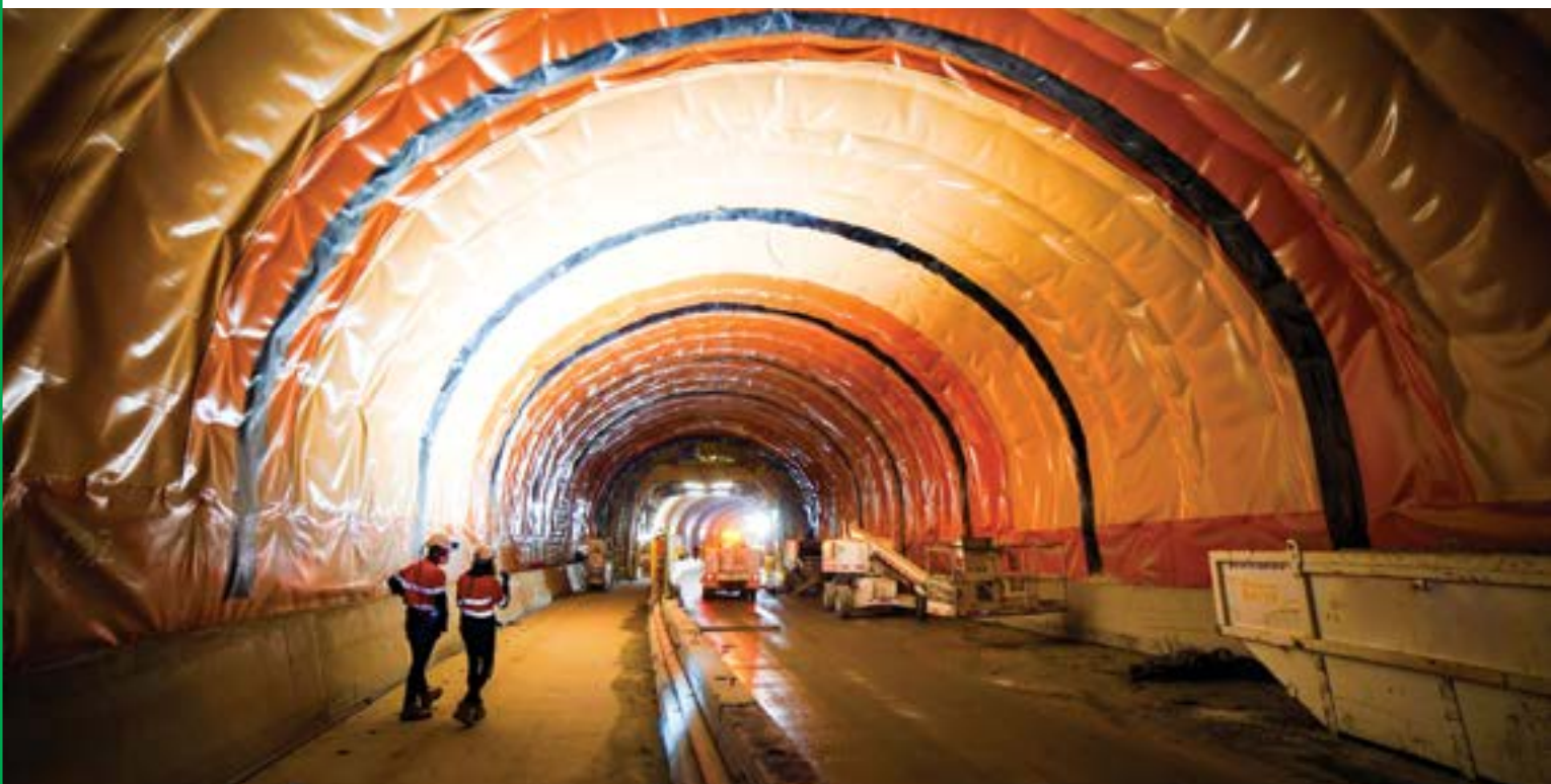
NorthConnex: final lining and waterproofing.
