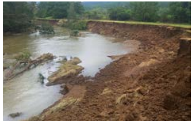
Oxley River with severe riverbank erosion.
