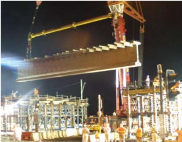
Night works: Erection of the bridge girders over Weakleys Drive Interchange, June 2008.
