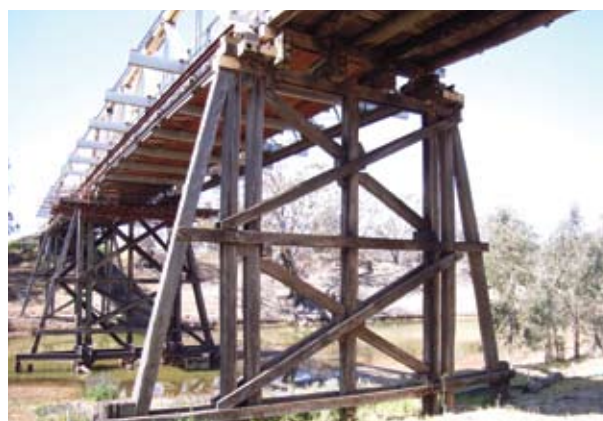
Coonamit Bridge, Wakool.
