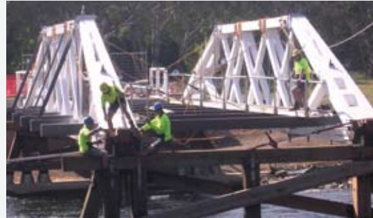
Restoration works on Junction Bridge, Tumut.
