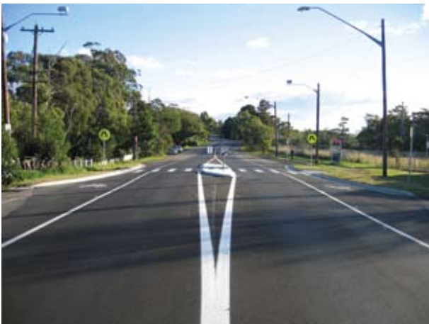
Pacific Highway near Cowan in Northern Sydney: The Pedestrian improvements narrowed the road into a single lane to force drivers to proceed with greater caution. It also improved the pedestrian footpath around the crossing.
