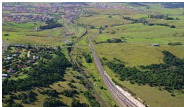
Aerial view of Oaks Flats to Dunmore.
