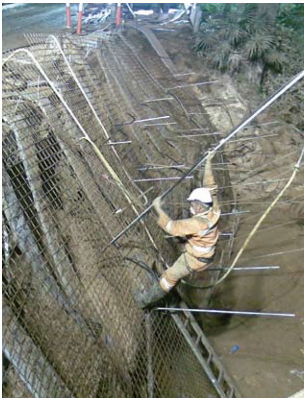
Maintenance engineer from Southern region repairing road damage at Bulli Pass.
