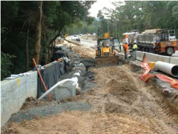
Central Coast Highway, upgrade work.
