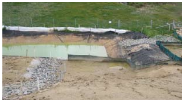
Sediment basin, Cooperook to Herons Creek upgrade.
