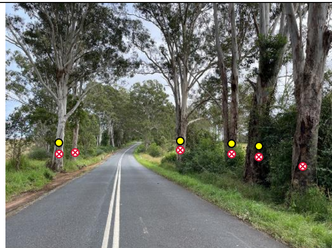
Plate 12: Eastern extent of tree removal looking west. Most trees within 9m of centre line are proposed to be removed.
