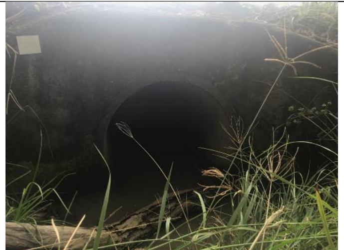
Plate 4: Single pipe culvert 516268, 380m west of Little Creek, is proposed to be extended or replaced with a new structure. The presence of deep cracks between pipe sections provides low to moderate value bat habitat; however, no indication of bat habitation was found during surveys. Shallow standing water was present on the 3 rd of May 2022.
