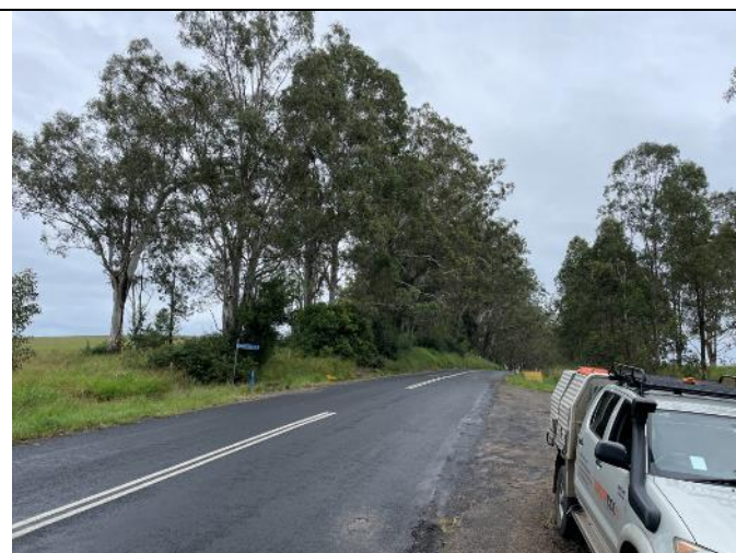
Plate 14: View west from Dump Road and Bruxner Highway intersection. All but five (5) trees upon the bank on the southern side of the highway are to be retained from Dump Road to Sandilands Rest Area.
