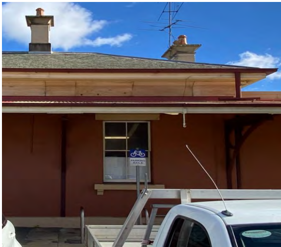
Figure 5.56 Room A4—East Elevation.
