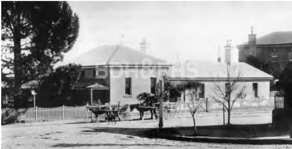
Figure 2.5 Old Court House and Police Station, Moss Vale, NSW, 1900s. This image shows the north elevation of the old Court House and police station in Bay Street. In the background is the two-storey railway station building. (Source: Berrima District Historical & Family History Society Inc)
