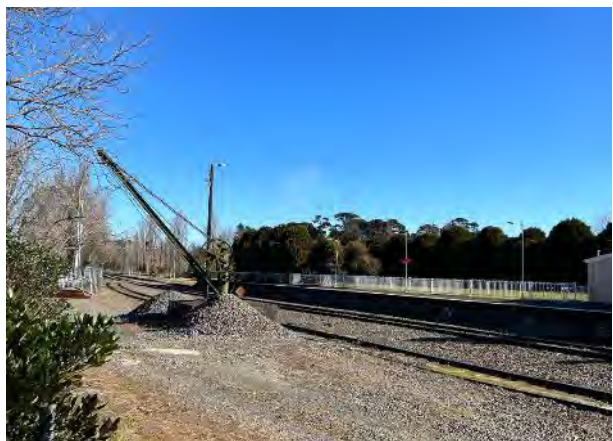
Figure 4-44: Jib crane looking southwest toward Platform 2 from Argyle Street footbridge (AECOM, 2023)
