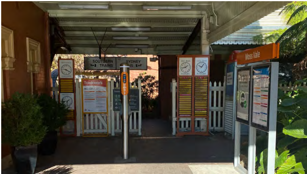
Existing timber gate west of the booking office. (Source: GML April 2023)
