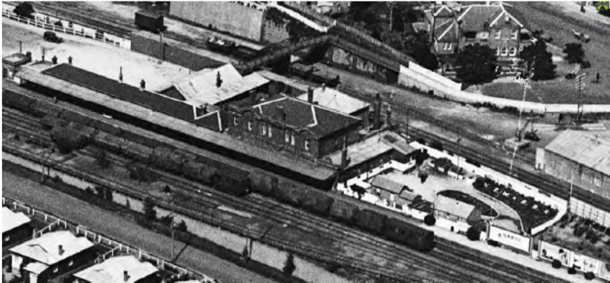
Figure 3-14: 1930s aerial view of Moss Vale Railway Station (VPR)
