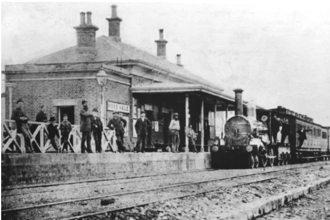
Figure 3-6: Moss Vale Railway Station, c. 1880 (Berrima District Historical and Family History Society in OCP Architects, 2020:17)
