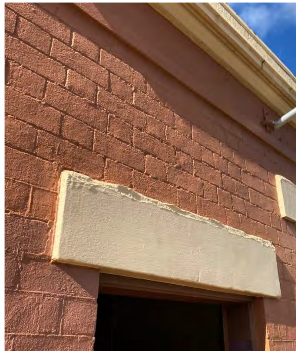
Figure 5.36 Header of Room D22.
