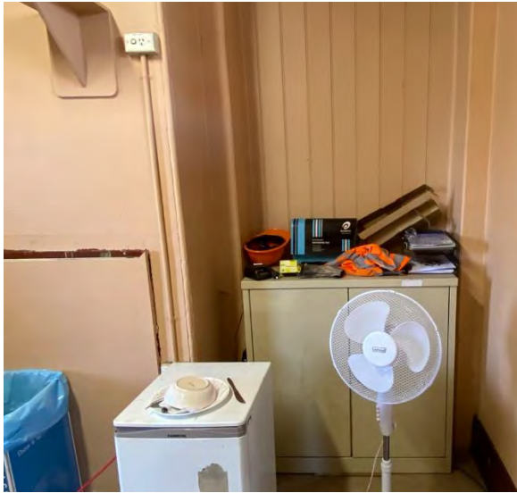
Figure 5.68 Room A4 – East Wall Lower.
