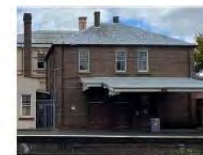
1. Two Storey Accommodation Addition - Looking West
