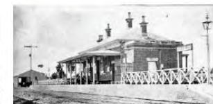
4. Original Station - Looking North
