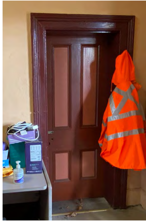
Figure 5.88 Room A5 – North Elevation.
