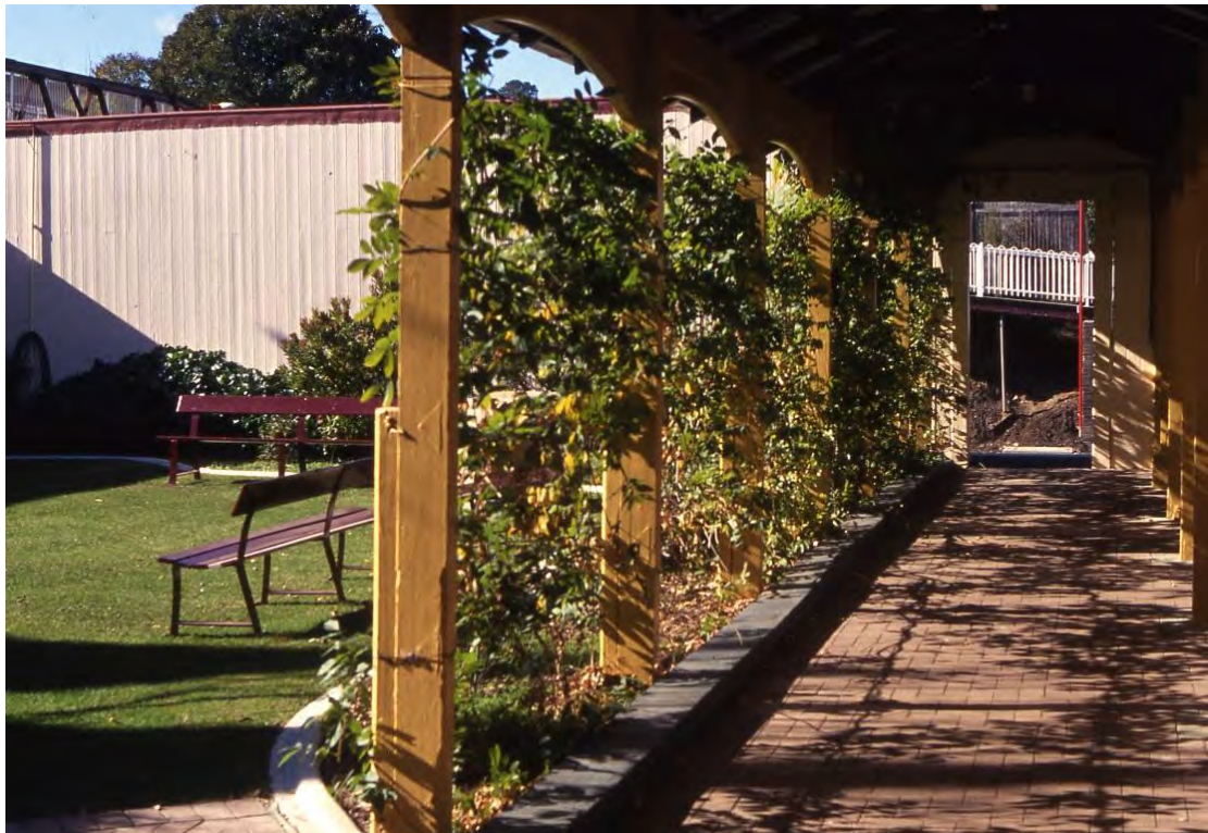
Figure 4.17 A similar eastern view of the Courtyard Garden in 1994 showing the wisteria vine, extensive pruning and remodelling of the garden beds. (Source: ARHS, provided by TfNSW)
