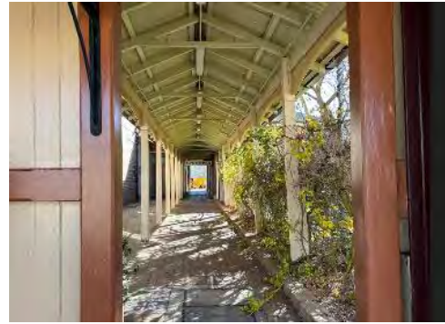
Figure 4-17: Breezeway looking west from Platform 2 to Platform 1. The wisteria boundary of the courtyard can be seen at right and building B at left (AECOM, 2023)
