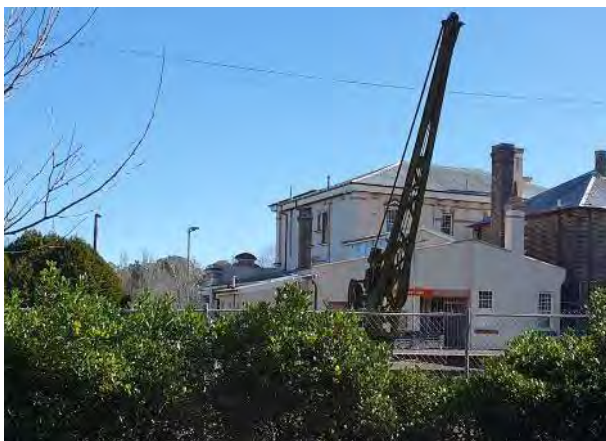
Figure 4-43: Jib crane (c.1884) as seen from Railway Street, looking west (AECOM, 2023)
