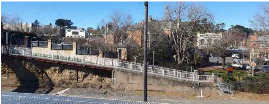
Figure 4-25: Ramp to Argyle Street looking east (AECOM, 2023)
