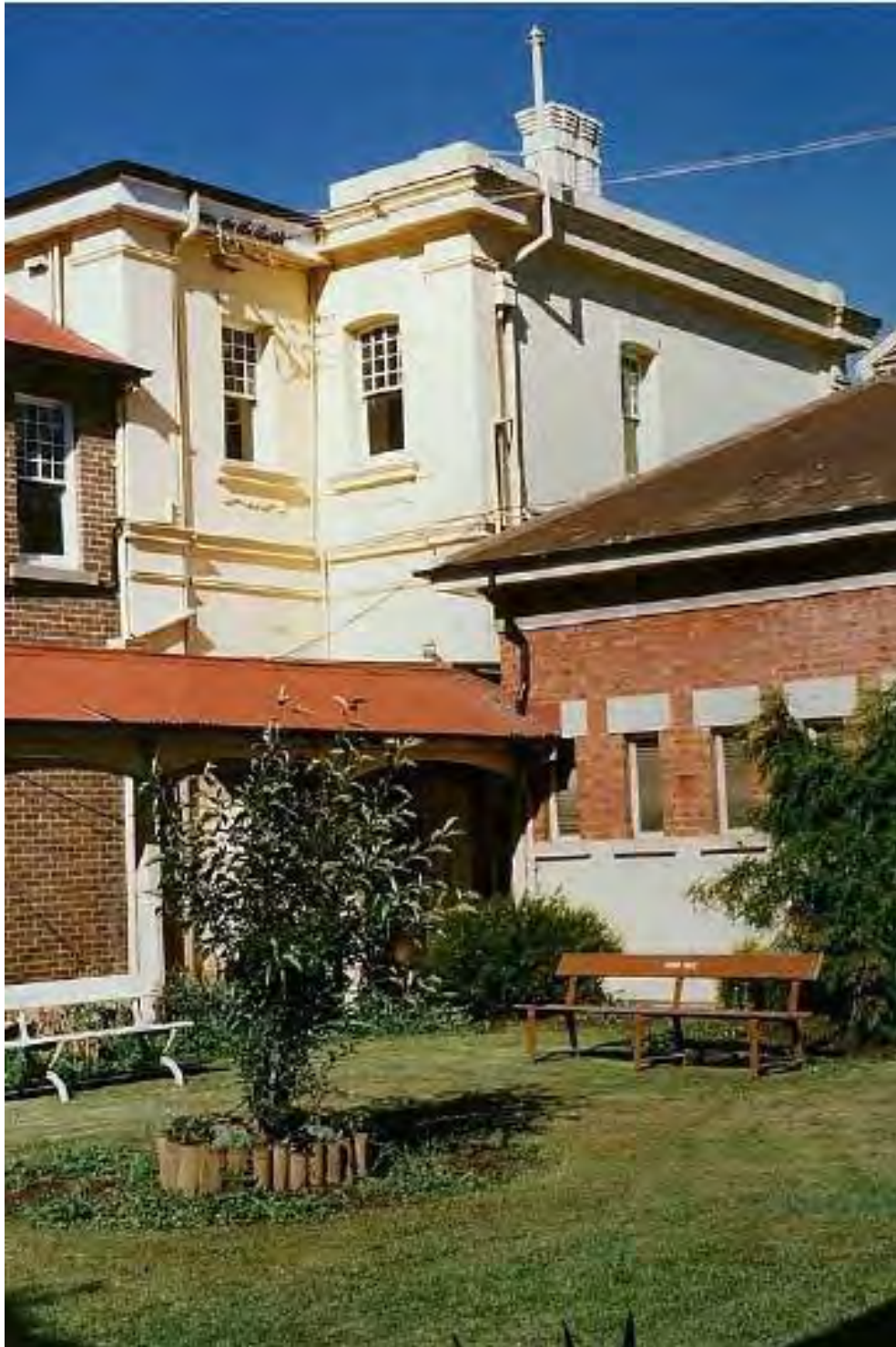
Figure 4.14 Moss Vale Station Gardens, 27 January 1987 showing the Courtyard Garden with little attention to detail or maintenance, with historically inappropriate treated pine vertical edging to the shrub in the lawn. (Source: CMP 2020)
