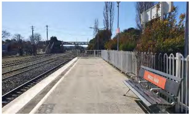
Figure 4-37: Platform 1, looking north, with Lackey Road footbridge in centre (AECOM, 2023)
