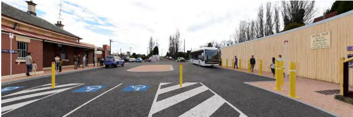
Figure 8-6: View after proposal from Moss Vale Railway Station looking north along Dalys Way (Source: AECOM)
