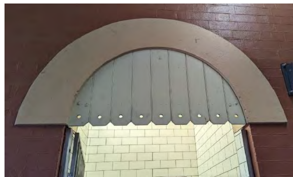
Figure 5.119 Room A17-D13-Rendered Arch and timber fretwork.
