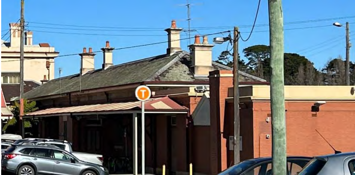
Figure 4-6: Building A, looking southwest (AECOM, 2023)
