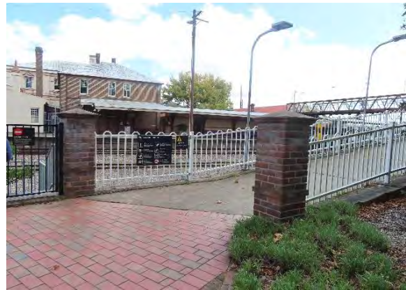
Figure 5.28 View of the brick piers and ramp leading to the Argyle Street footbridge, looking north from Jubilee Park.
