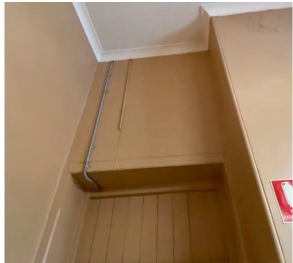
Figure 5.63 Room A4 – East Wall Upper.
