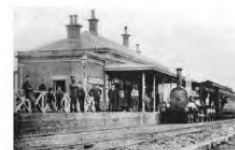
3. Original Station - Looking South
