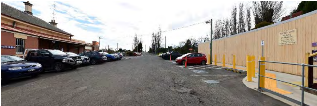
Figure 8-5: Existing view from Moss Vale Railway Station looking north along Dalys Way (Source: AECOM)
