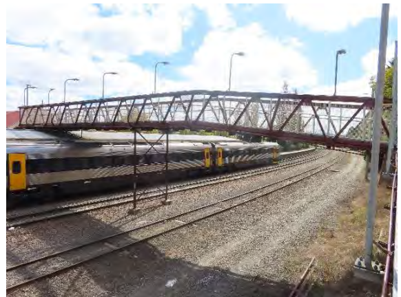
Figure 5.24 View of the Argyle Street footbridge, looking west.
