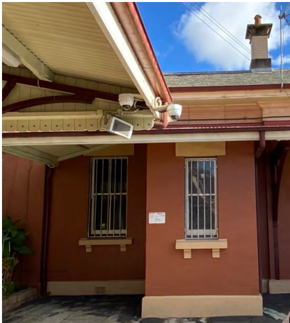
Figure 5.97 Room A9—East Elevation.
