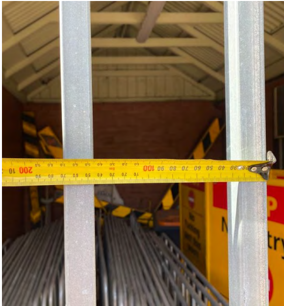
Figure 5.43 Room A2 – Aperture of grilles and roof structure.
