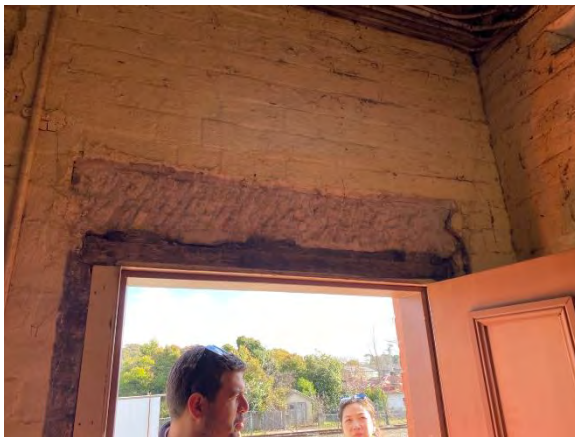
Figure 5.35 Room A1 – Lintel of door D22.
