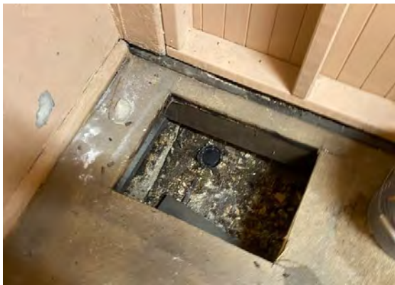
Figure 5.78 Room A4 – Later addition infill.
