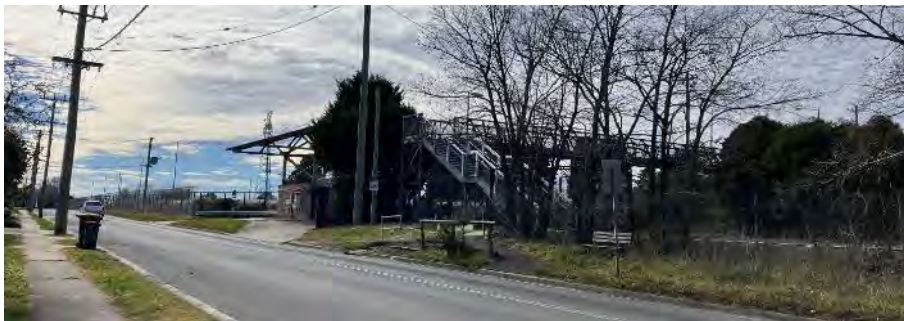
Figure 4-27: Lackey Road stair and footbridge looking north (AECOM, 2023)
