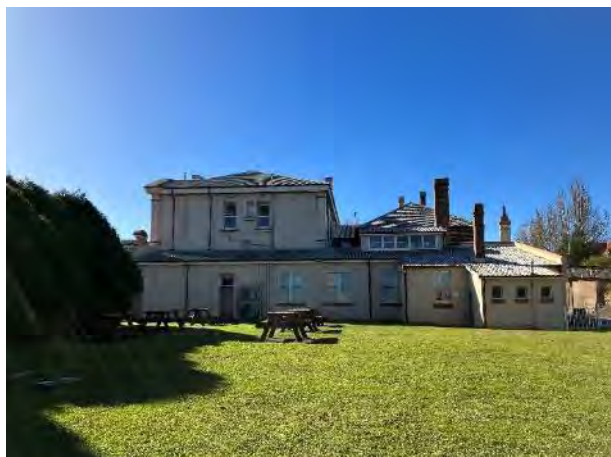
Figure 4-31: Refreshment Room Gardens looking north (AECOM, 2023)
