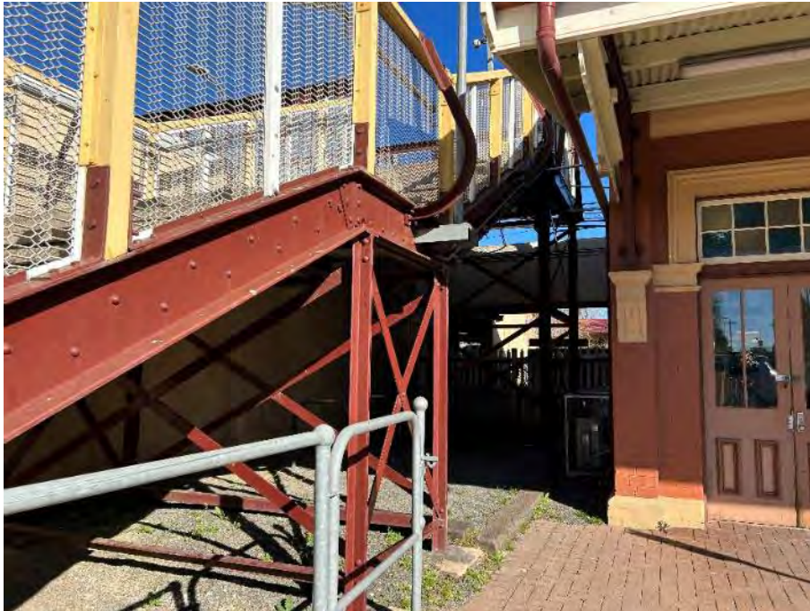
Figure 4-29: Stair to forecourt looking south (AECOM, 2023)
