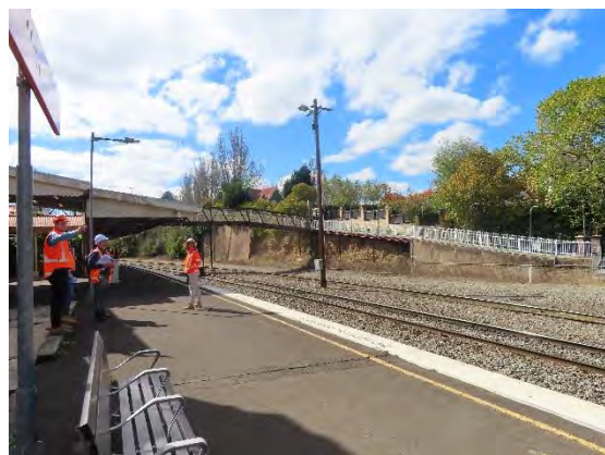
Figure 5.10 View of the eastern platform, looking north.
