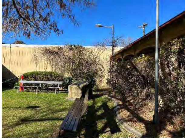
Figure 4-33: Courtyard looking south showing timber batten finish to platform awning (AECOM, 2023)
