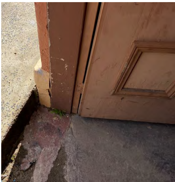
Figure 5.45 Room A1–Sill of door D22.
