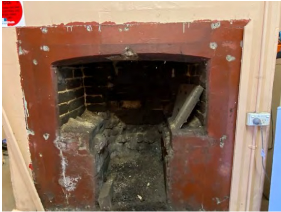
Figure 5.60 Room A4 – Fireplace.
