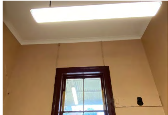
Figure 5.61 Room A4 – East Wall.
