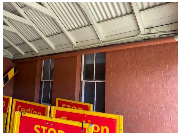
Figure 5.48 Room A3—North Elevation.
