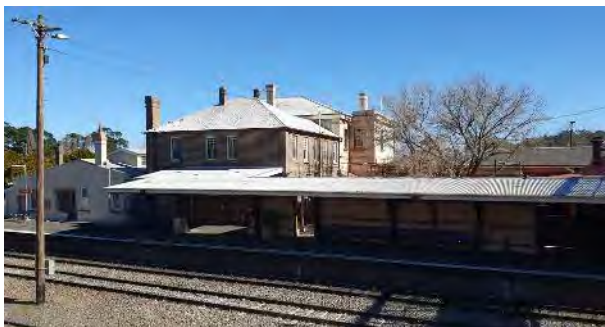
Figure 4-38: Platform 2 as seen from the Argyle Street footbridge, looking west. Building B including the former Refreshment Room is at left (AECOM, 2023)
