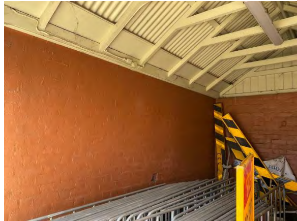
Figure 5.44 Room A2 - South Elevation.
