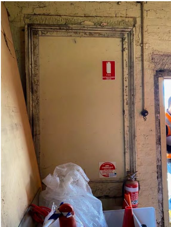
Figure 5.39 Room A1 – East elevation.
