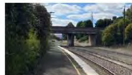
1. Dalys Way Bridge - Looking North
