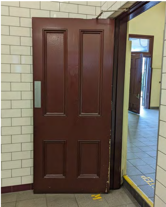
Figure 5.114 Room A13-D23—Outside Face.
