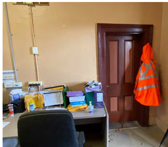
Figure 5.75 Room A4 – South Wall Lower.
