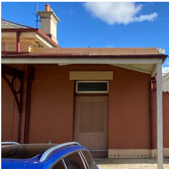
Figure 5.47 Room A3—East elevation.
