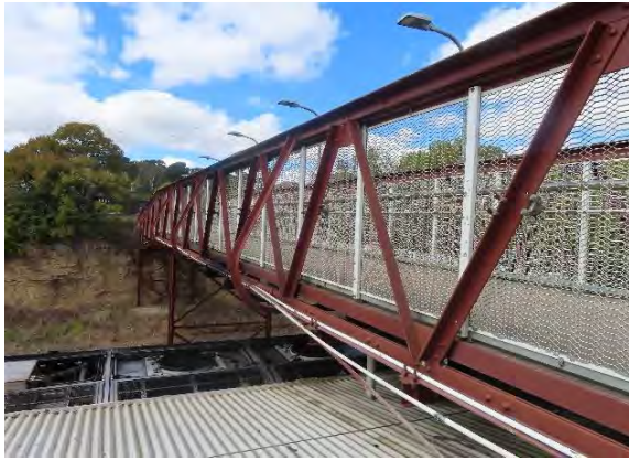
Figure 5.25 View of the Argyle Street footbridge and embankment, looking east.
