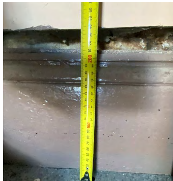
Figure 5.82 Room A5 – Skirting Profile.
