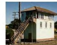
5. Signal Box - Looking North-west
