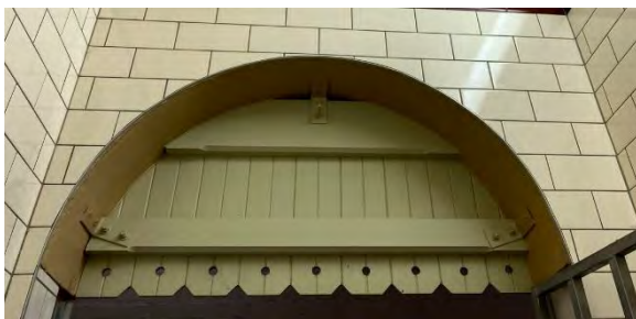
Figure 5.120 Room A17-D13-Timber fretwork.
