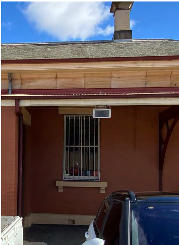
Figure 5.81 Room A5 – East Elevation.
