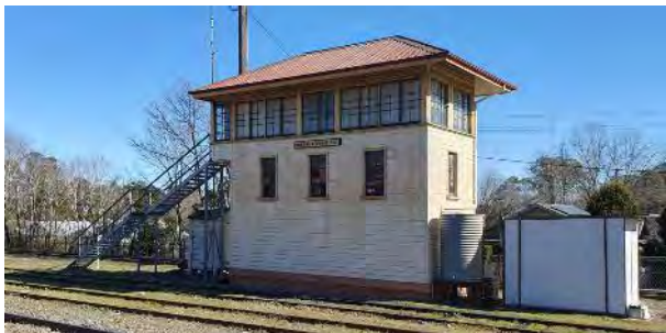
Figure 4-41: Signal box (1915) (AECOM, 2023)
