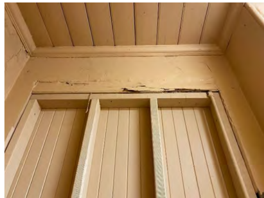
Figure 5.79 Room A4 – Later addition infill.
