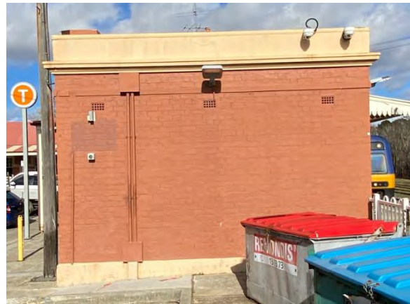
Figure 5.34 North elevation of Room A1.
