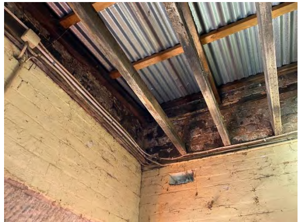
Figure 5.40 Room A1 – Ceiling looking northwest.
