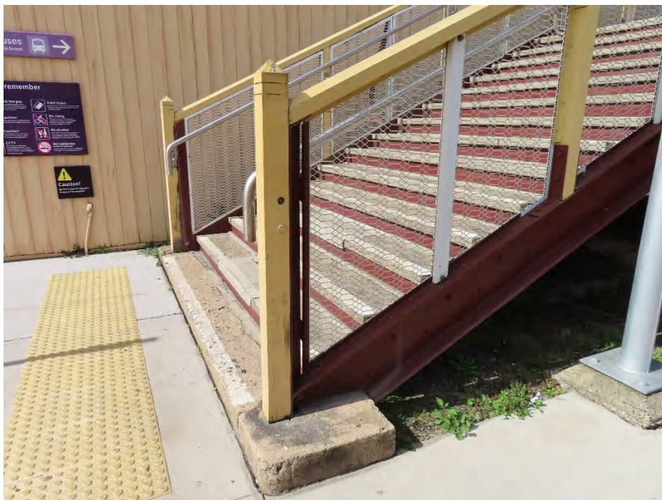
Figure 5.20 Reconstructed timber posts and rail along the stairway. (Source: GML 2023)
