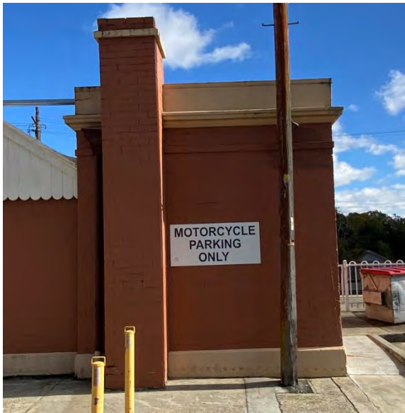
Figure 5.33 East elevation of Room A1.
