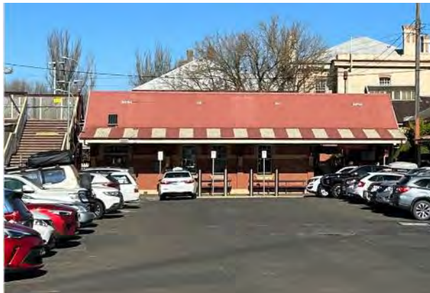
Figure 4-18: Building C looking south from the station's forecourt/car park. The steps to the Argyle Street footbridge are at left, and the Governor's Rooms of Building B at right (AECOM, 2023)
