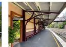
4. Down Platform and Awning - Looking North
