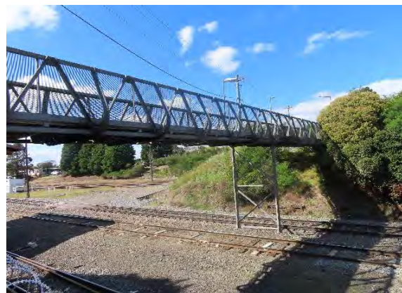
Figure 5.31 View of the footbridge along Lackey Road, looking east.
