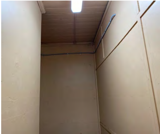
Figure 5.76 Room A4 – Rear of fireplace – Looking west.
