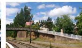
3. Footbridge No 2 (South) - Looking North
