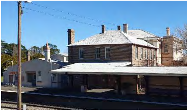
Figure 4-16: Building B, looking west from Argyle Street footbridge (AECOM, 2023)
