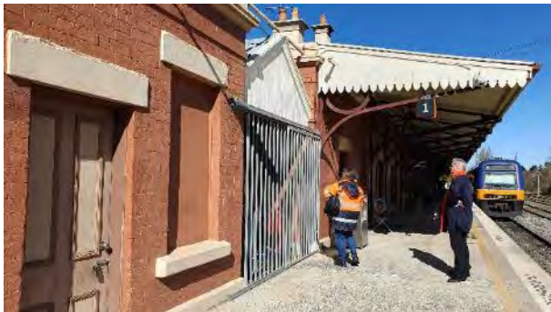
Figure 4-7: A2 Shelter Room, Building A (AECOM, 2023)
