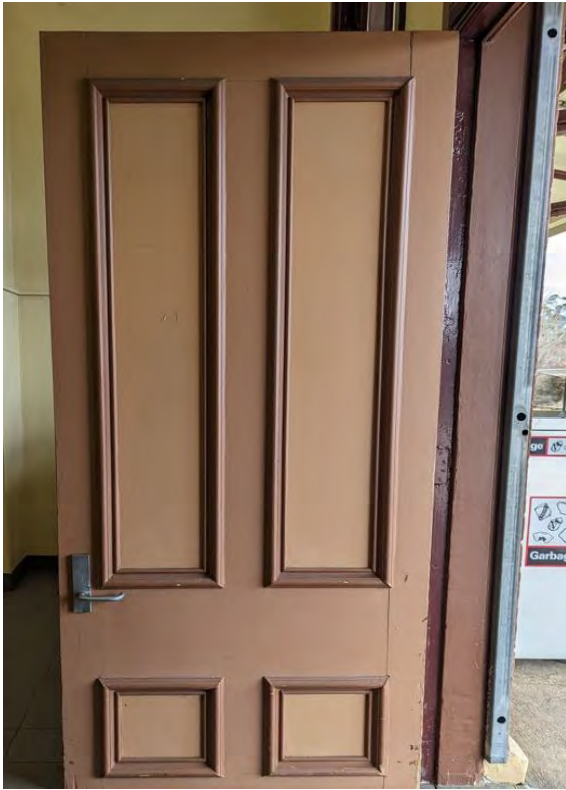
Figure 5.112 Room A13-D15—Outside face.
