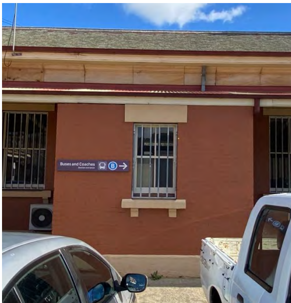
Figure 5.91 Room A6/A7—East Elevation.
