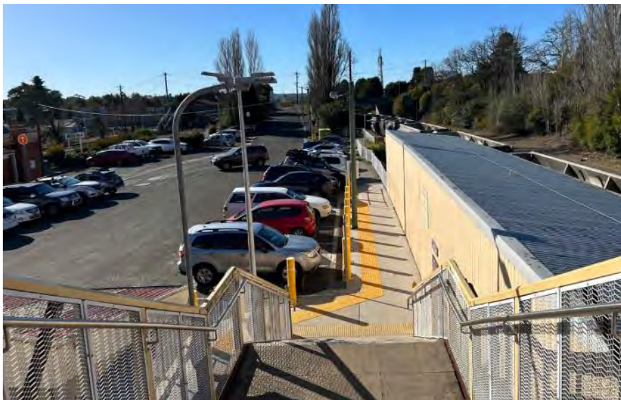
Figure 4-28: Stairs leading from Argyle Street footbridge to the station's forecourt. Building C is at left, and Platform 2 is at right (AECOM, 2023)
