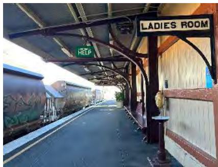
Figure 4-39: Platform 2 looking south (AECOM, 2023)
