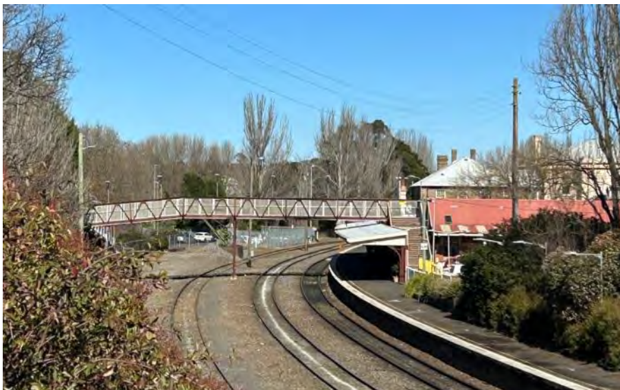
Figure 4-22: Argyle Street footbridge, looking south from Dalys Way overbridge (AECOM, 2021)
