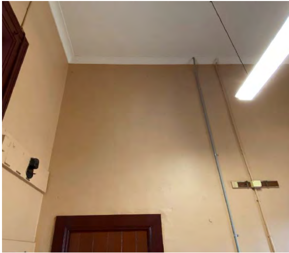
Figure 5.72 Room A4 – South Wall Upper.
