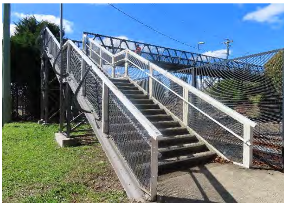
Figure 5.30 View of the stairway to the footbridge along Lackey Road.
