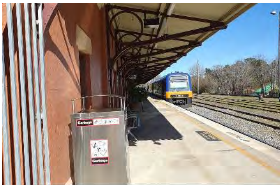
Figure 4-36: Platform 1, looking south (AECOM, 2023)
