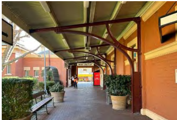
Figure 4-19: Breezeway between Platforms 1 and 2, looking west from Platform 2. The courtyard and the east-west range of building A can be seen at left, and the southern elevation of Building C at right (AECOM, 2023)
