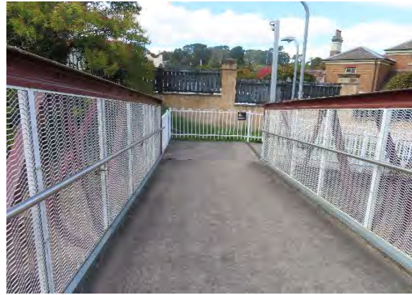
Figure 5.26 View of the Argyle Street footbridge, looking east.
