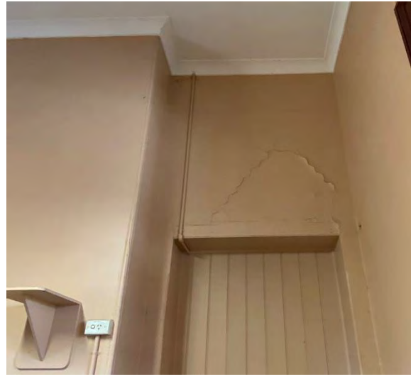
Figure 5.65 Room A4 – East Wall Upper.
