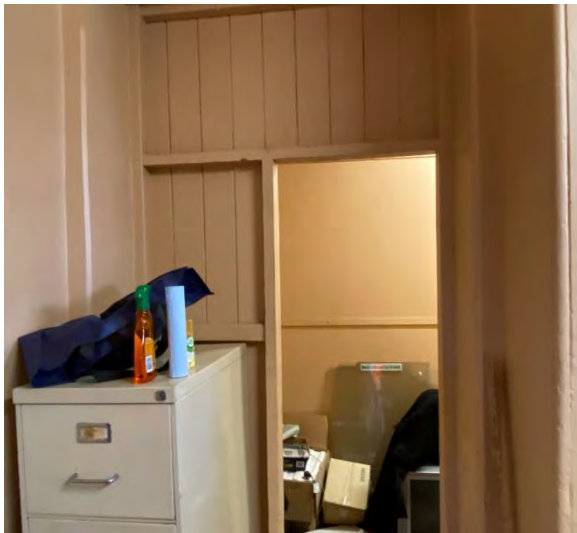
Figure 5.66 Room A4 – East Wall Lower.
