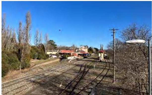
Figure 4-4: View of station from Lackey Road footbridge (AECOM, 2023)
