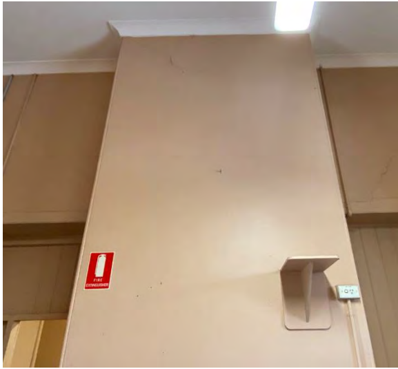
Figure 5.64 Room A4 – East Wall Upper.
