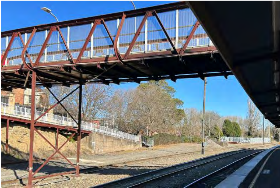
Figure 4-23: Argyle Street footbridge and ramp looking southeast from Platform 2 (AECOM, 2023)
