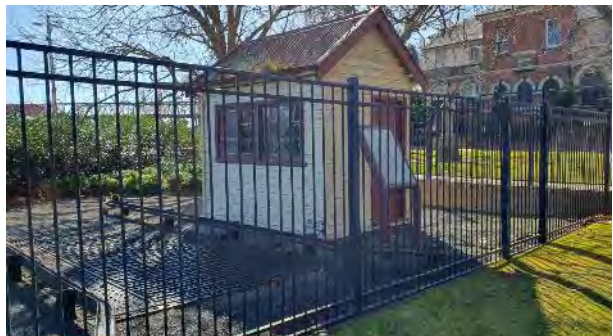
Figure 4-42: Weighbridge (c.1940s/1950s) on the eastern side of the station (AECOM, 2023)
