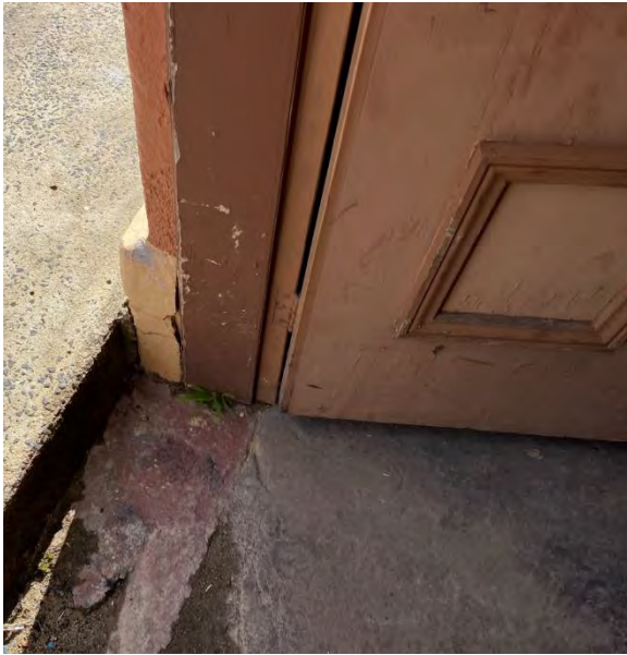
Figure 5.37 Room A1—Sill of door D22.
