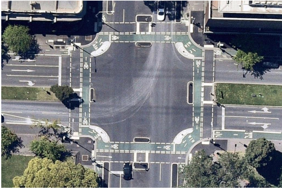
Figure 17. Protected intersection in East Melbourne, Victoria. Image credit: Nearmap.com
