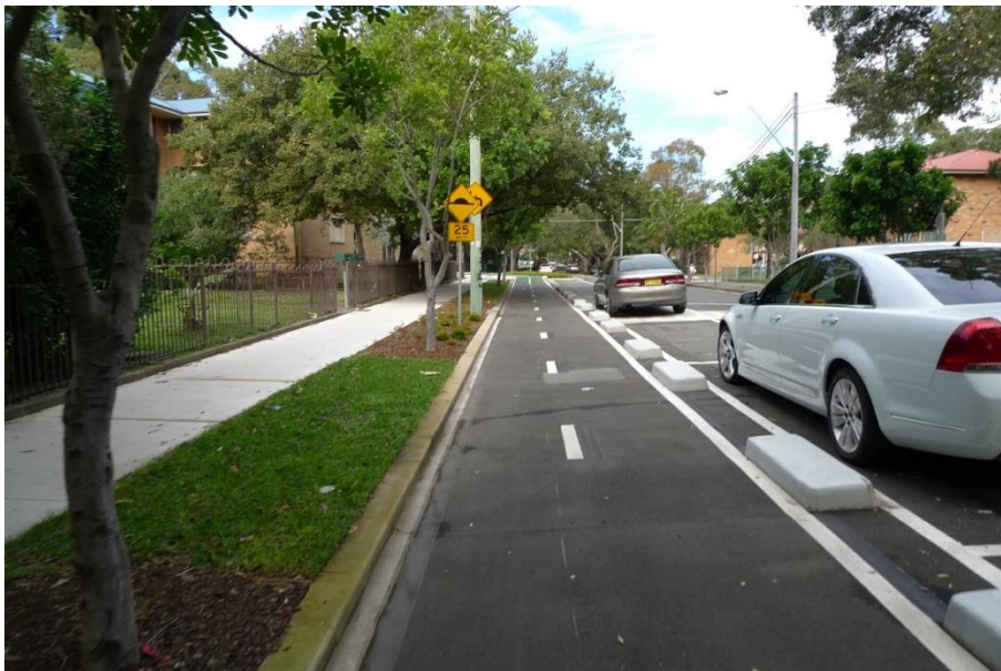
Figure 6: A hybrid design was used for the George Street cycleway. The southern section uses an intermittent median design to simplify construction and reduce costs. The medians are located to allow car doors to open between them – this required marking the parking bays. Image credit: Warren Salomon.
