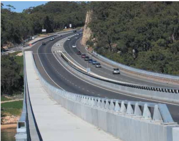
Alfords Point Bridge, opened to traffic in August 2008.
