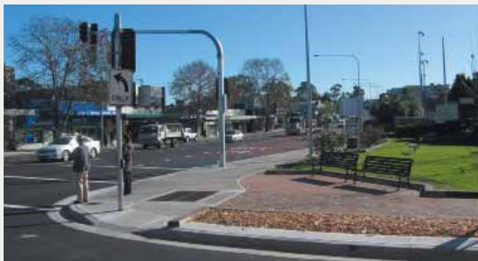
Bus priority project at the intersection of Old Northern Road and Windsor Road, Baulkham Hills, Sydney.
