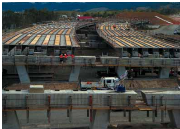
Construction works showing the placement of pre cast super-t girders on the Teven Road Bridge (360m in total length).
