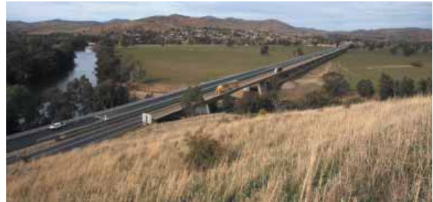
View of the duplicated Sheahan Bridge, Hume Highway, Gundagai.
