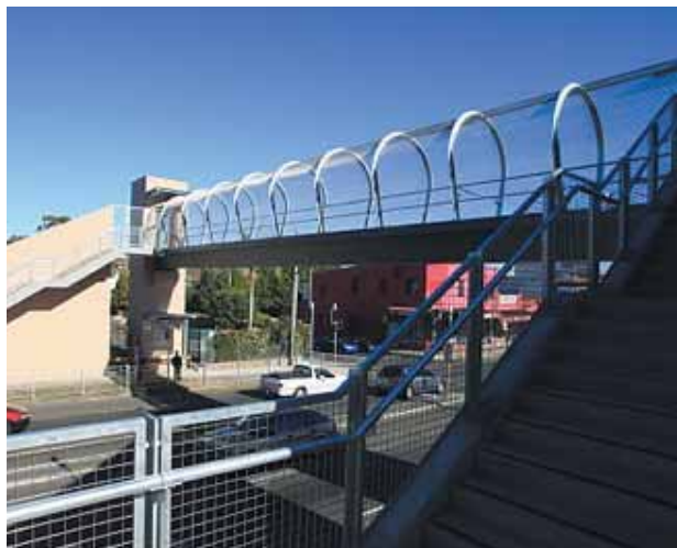
New Haberfield pedestrian bridge.
