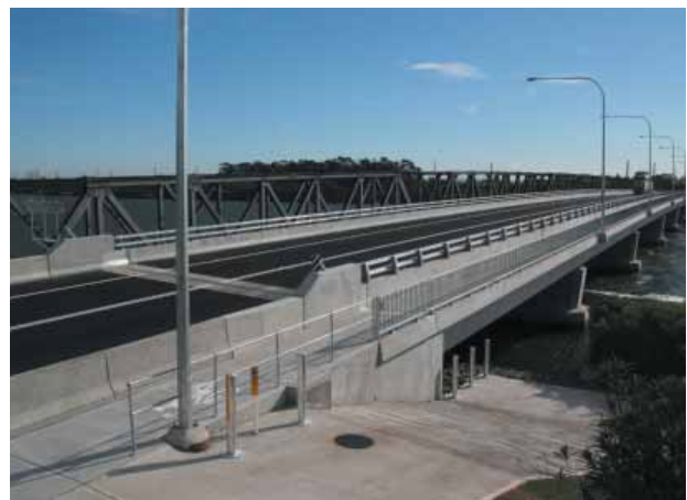
The new Tourle Street Bridge alongside the original steel truss bridge.
