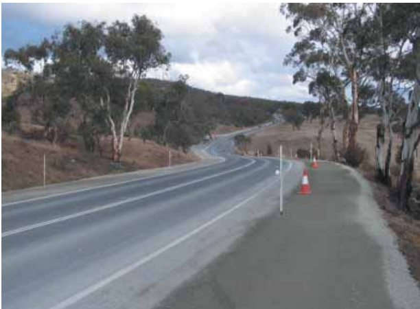
Shoulder widening along the Kings Highway.
