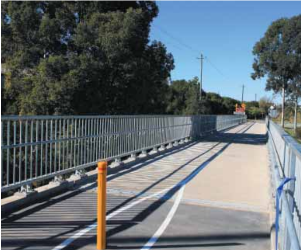
Footbridge and cycleway over the Wianamatta Creek, Windsor.
