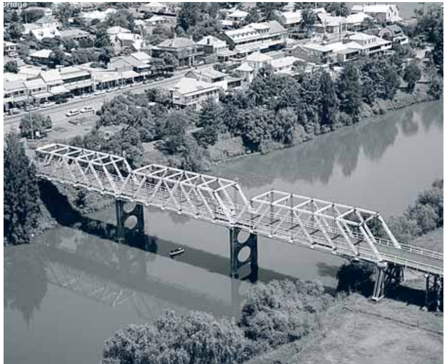
The NSW Heritage Council has approved emergency works to historically significant Morpeth Bridge, one of only three similar structures remaining in the State.
