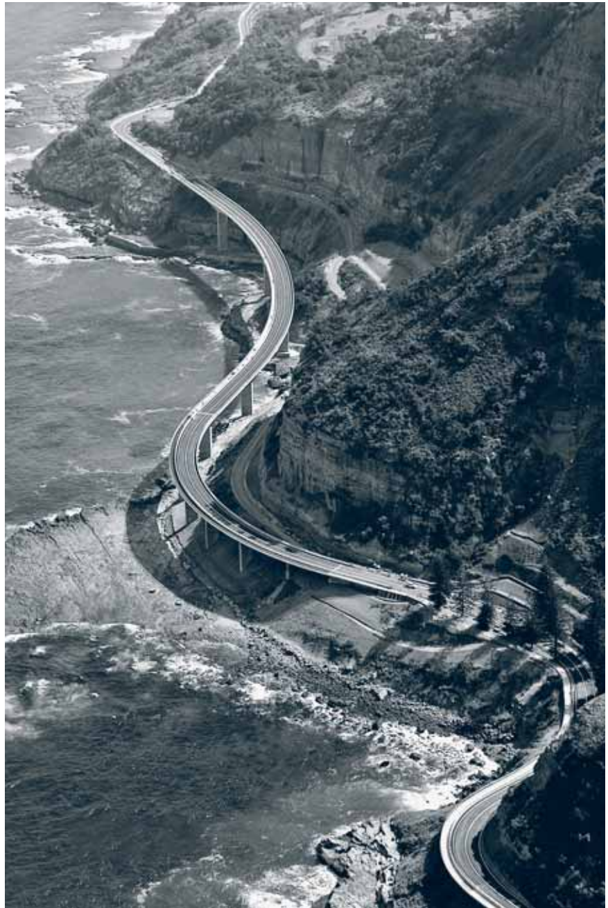
The flowing design of the recently opened Sea Cliff Bridge on Lawrence Hargrave Drive fits into its setting and offers road users a unique experience.
