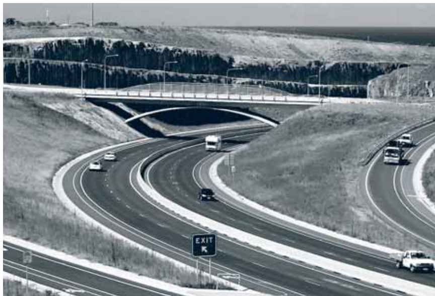
The Bombo Interchange at the North Kiama Bypass was completed and opened to traffic in November 2005.
