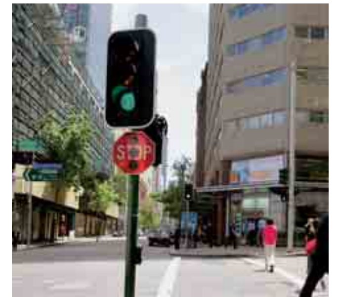
LED lights have been installed at the corner of Kent and Market streets in Sydney, the site of Sydney's first set of traffic lights in 1933.
