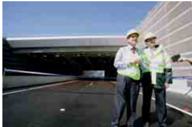
The Member for Riverstone John Aquilina and the Hon. Eric Roozendaal, Minister for Roads, opening the $40 million underpass at the intersection of Old Windsor Road and Norwest Boulevard.
