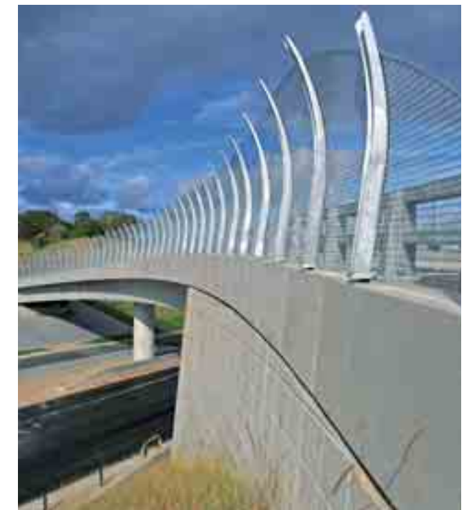
The opening of the Pacific Highway upgrade from Brunswick Heads to Yelgun, means 60 kilometres of the highway from Ewingsdale to the Queensland border will be uninterrupted dual carriageway.
