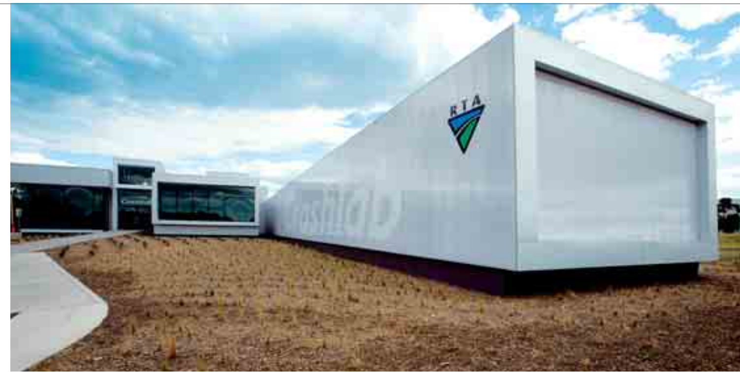
The RTA Crashlab, located at Huntingwood, delivers positive road safety outcomes through world-class testing of vehicles, crash barriers, safety harnesses and roadside furniture. Featured in the facility on the chapter page is the Hon. Eric Roozendaal, Minister for Roads.
