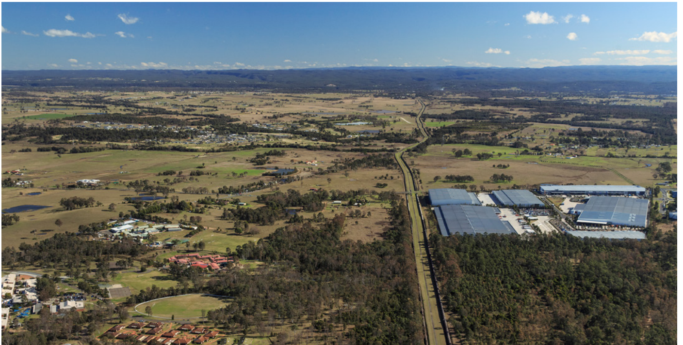
Looking west over Erskine Park and the Warragamba Pipeline towards Luddenham and Orchard Hills
