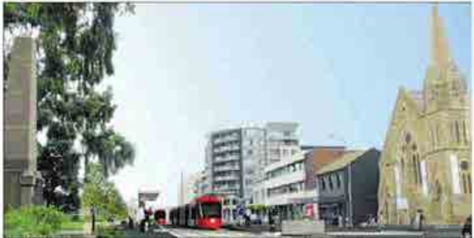
ALL ABOARD: Access to Parramatta Light Rail for an estimated 130,000 people within walking distance of stops will increase to 180,000 by 2041 – more than half of Parramatta's population. Stage one is due to be completed in 2023.
