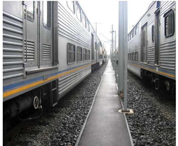
Upgraded Sidings 2 & 3 in Blacktown Stabling Yard
