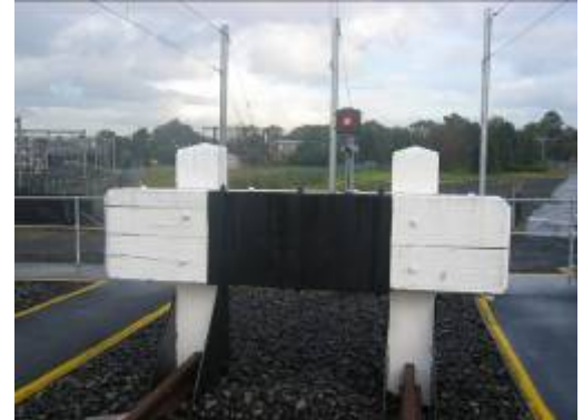
RailCorp Fixed Buffer Stop Type 204-88
