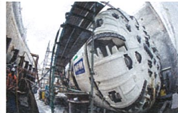
TBM3 Isabelle being assembled at Cherrybrook
