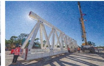
The launching gantry at Kellyville during the Italian Prime Minister's visit
