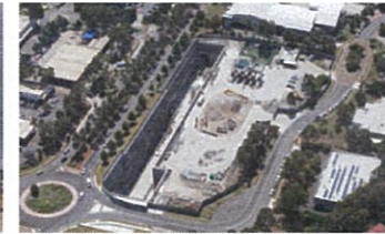
An aerial view of the Norwest Station site
