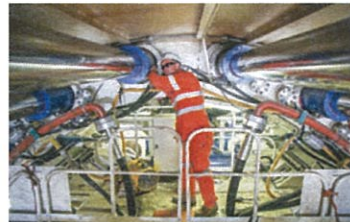
Performing maintenance on a TBM
