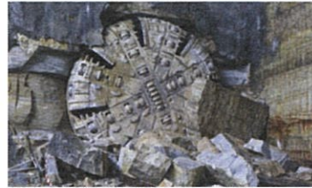
TBM2 Florence breaking through at Showground
