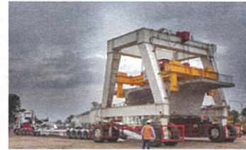
A straddle carrier lifts a skytrain concrete segment at Kellyville
